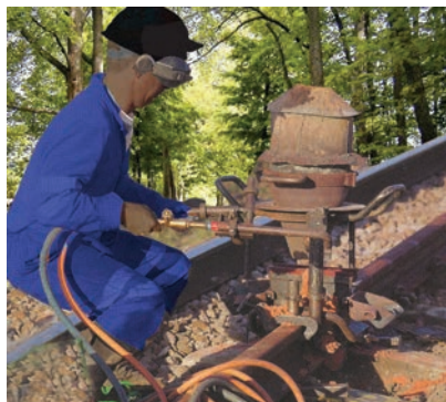
Figure 3.11 Thermit process for joining railway tracks
